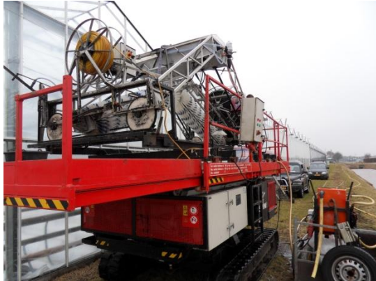
Img. 23 Roof cleaner on scissor lift
