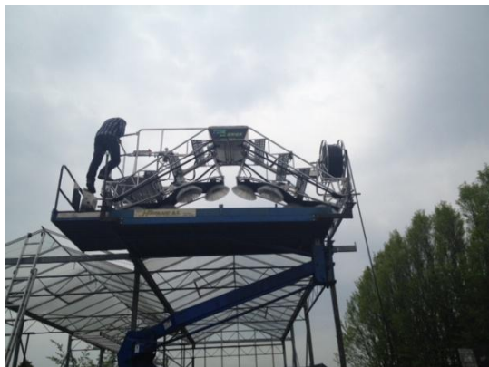
Img. 25 Roof cleaner on scissor lift
