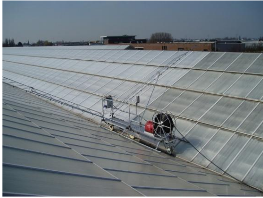
Img. 17 Chalking a wide peak of 12.80m
